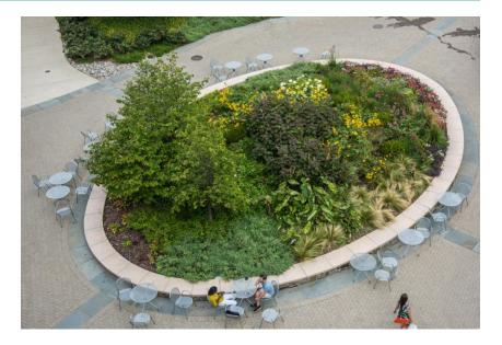
A green roof and a nearby bioswale reduce storm water runoff. Plants featured throughout the SIS landscape are local and adaptive species, and reduce the environmental impact of landscaping by thriving on less irrigation and requiring minimal use of pesticides and herbicides. A ground level green roof over underground parking and reflective white roofing help reduce the heat island effect, a phenomenon where urban areas experience warmer temperatures due to trapped heat.
