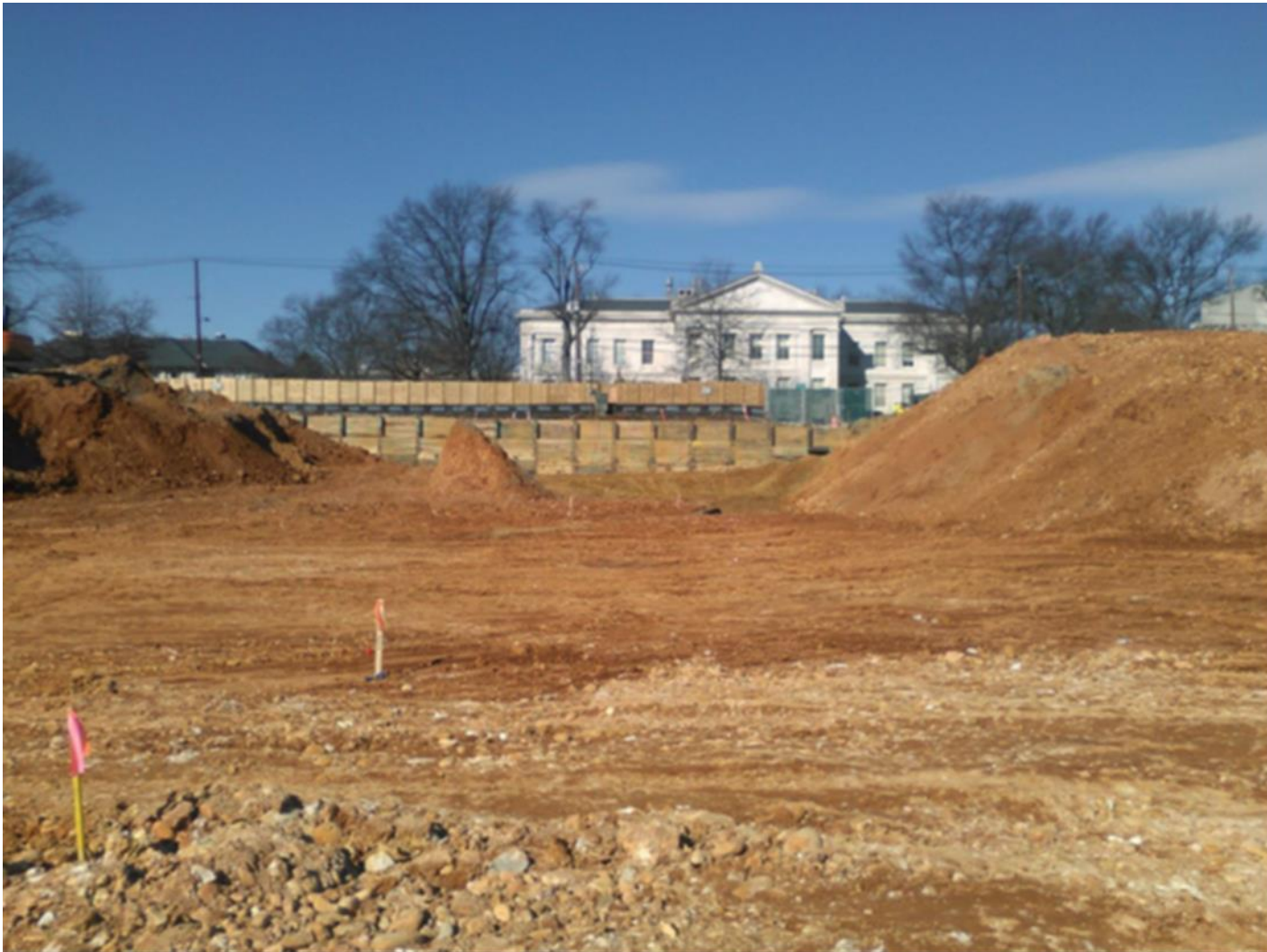
Garage excavation looking west
