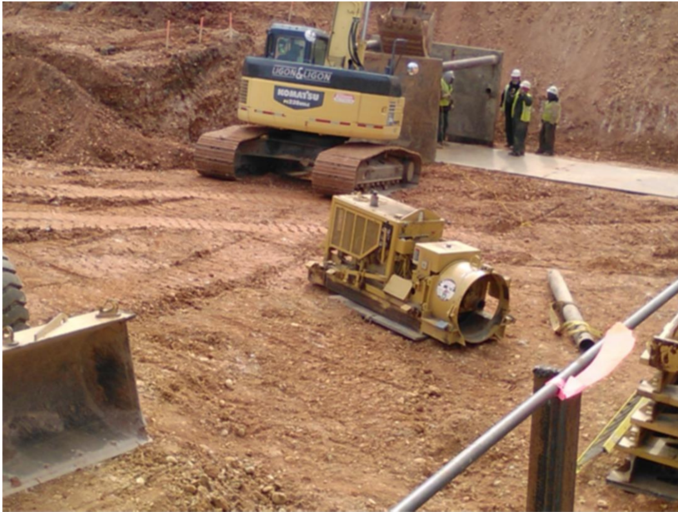
Excavation on Nebraska side of site
