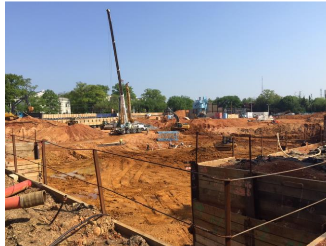
Garage excavation looking northwest
