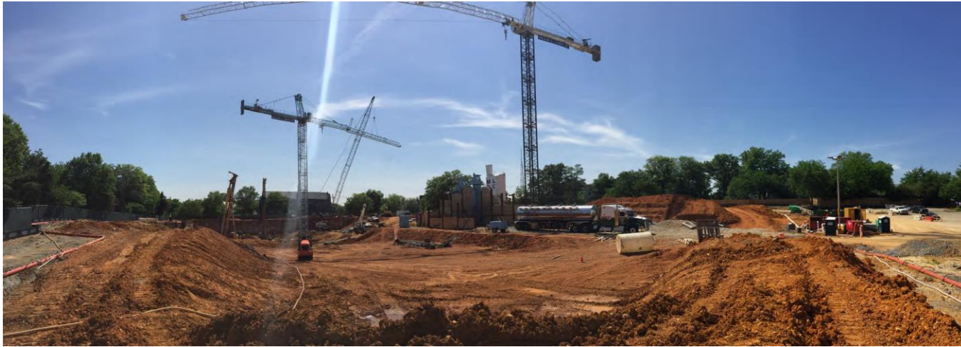
Garage excavation looking south
