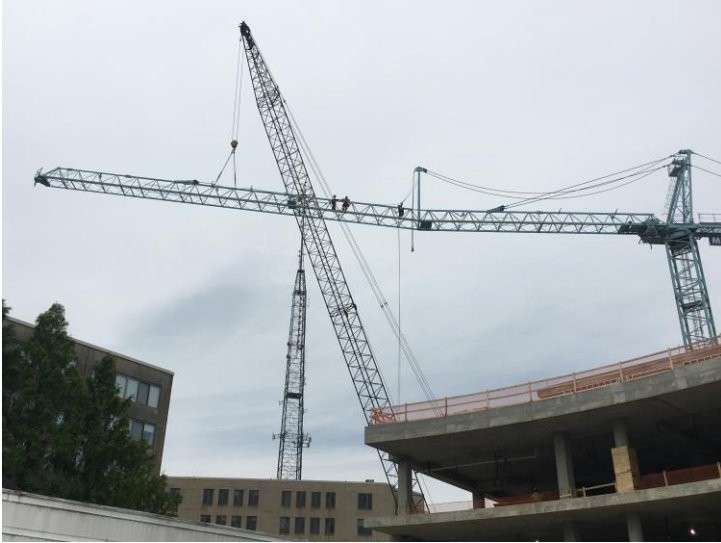
Tower crane removal
