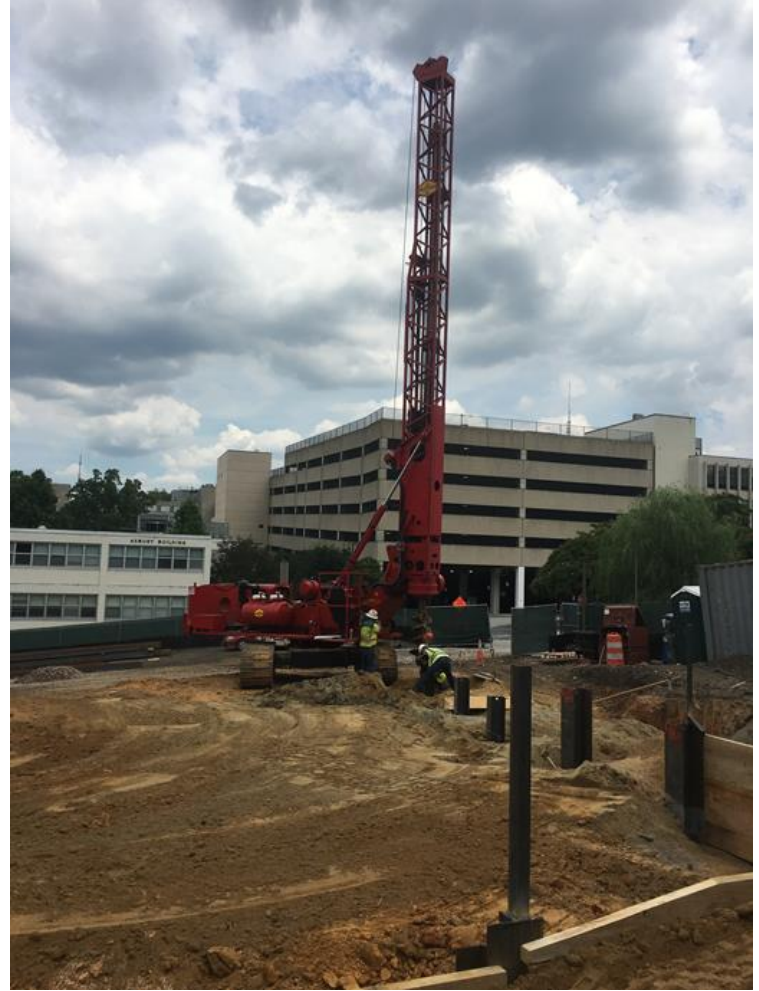
Soldier Pile Installation
