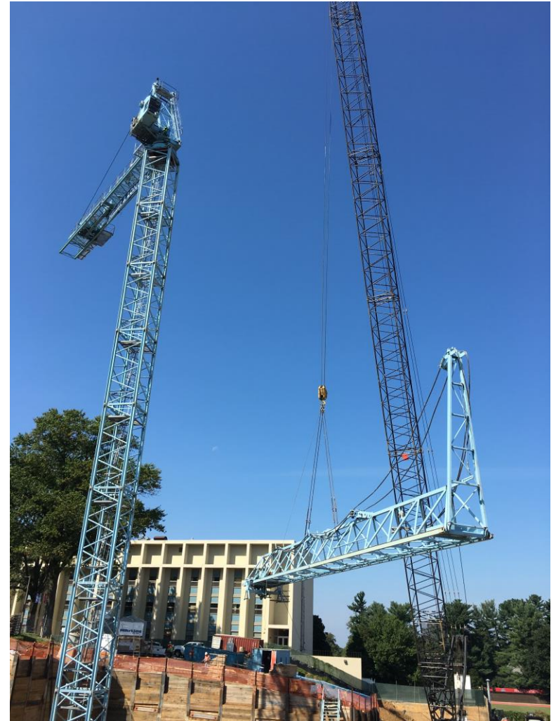
Crane Installation
