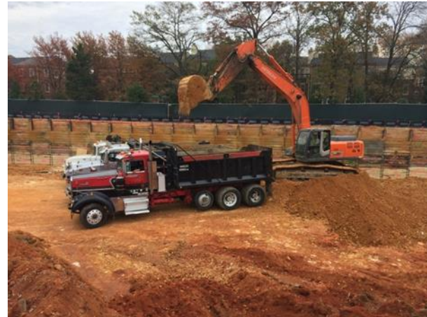
Lagging and Excavation
