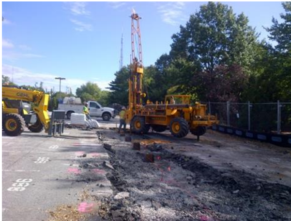
Dewatering System Installation
